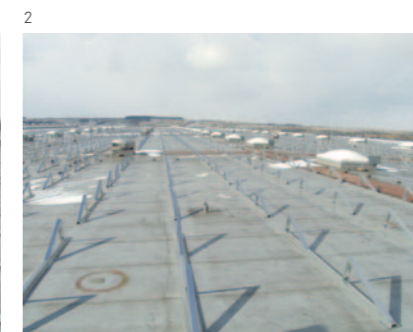
1 It took a total of just ten weeks to construct the Emsbüren facility, from planning to grid-connection.
